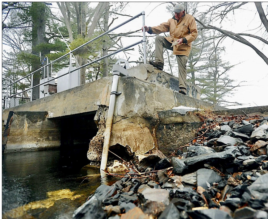
Dick Greenan, chairman of the Belgrade Lakes Watershed Dams Committee, checks out damage to the base of the Belgrade Village Dam in March. Repairs are expected by Nov. 1. Rich Abramson/Morning Sentinel photo (used with permission)
