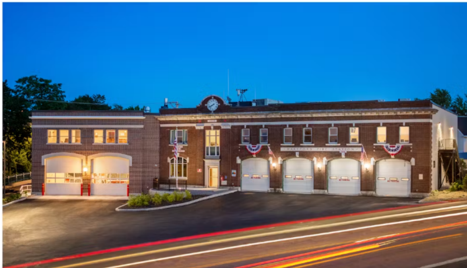
Hartford Fire Station, before (top) and after (bottom) the addition and renovation work NOD completed in 2019
