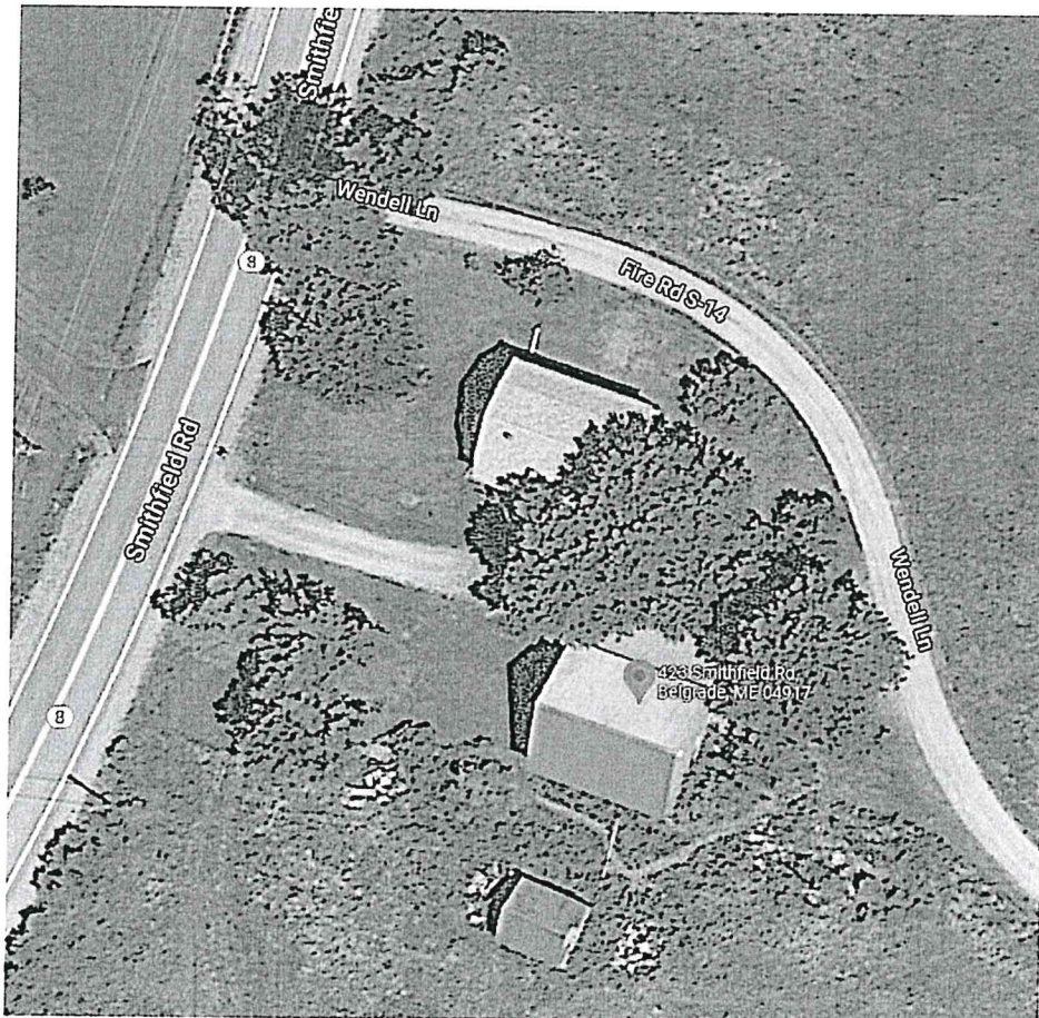
Aerial view of the site
