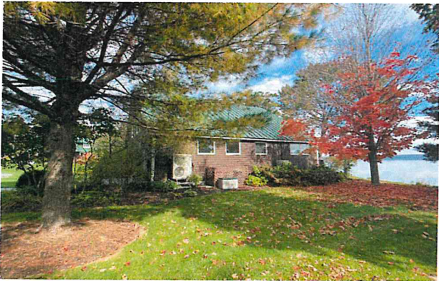
Existing cottage, south elevation
