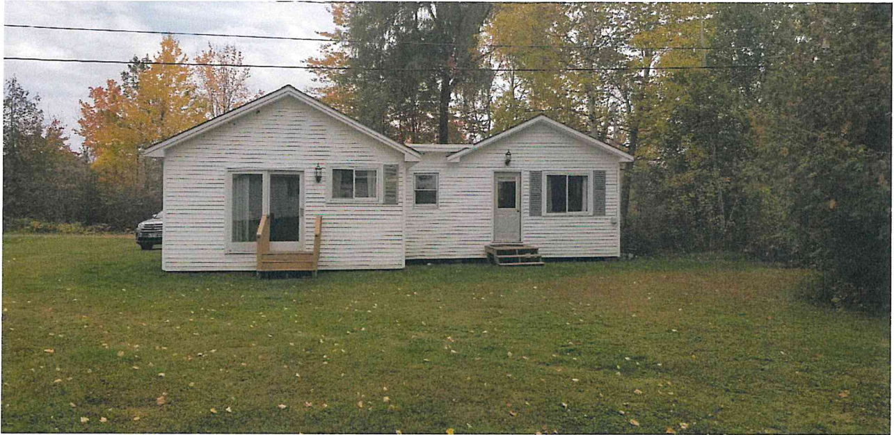
Photo 1: The front of the 2-bedroom camp closer to the road. Note the power lines that cross just in front of the building.
