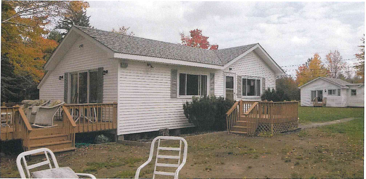
Photo 5: A side view of the existing structure that is closer to the shoreline. The rear camp can also be seen to the right.
