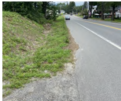
Drainage swale along Rt. 27 and Self-Storage Lot facing north
