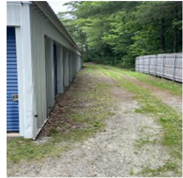
Fence along south property line
