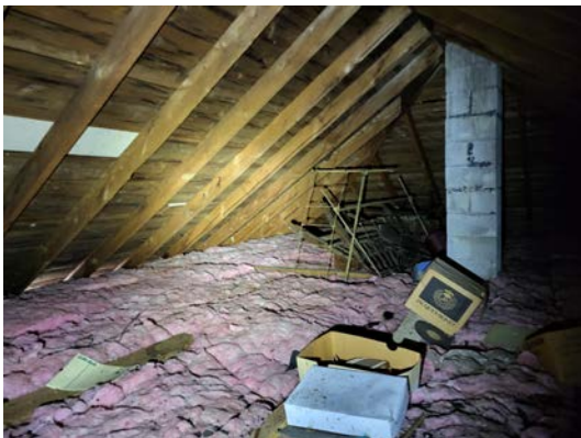
General view of Attic
