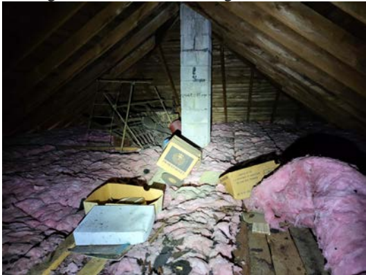
General view of Attic
