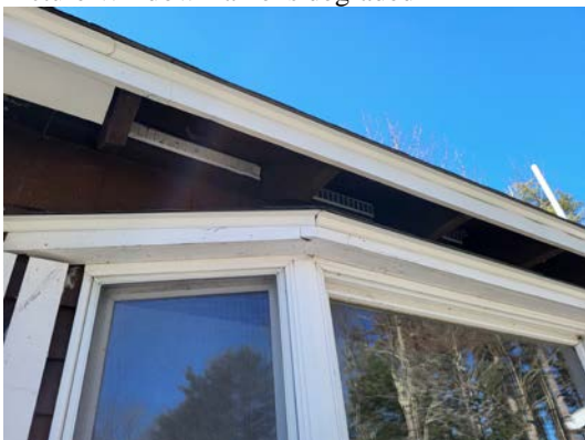
View of soffit vents
