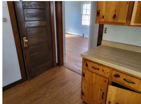
View of door to Basement
