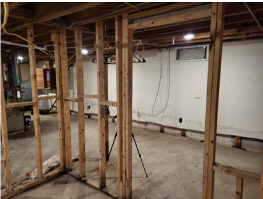
General view of Basement
