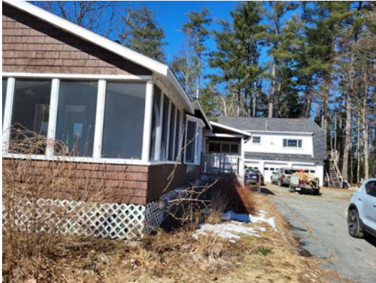
No gutter on this roof line
