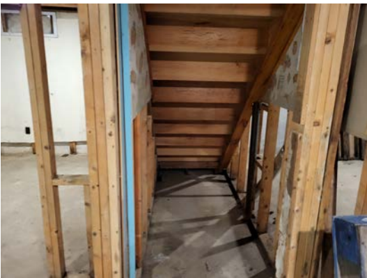
General view of Basement
