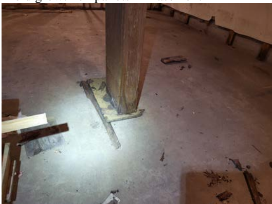
Raised floor fragment remain in Basement
