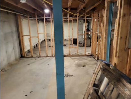
General view of Basement
