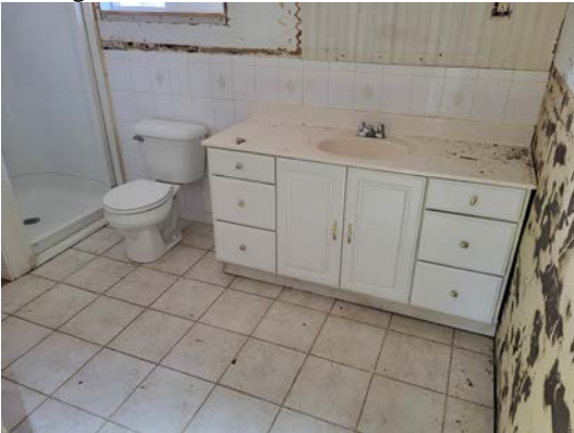
View of Bathroom
