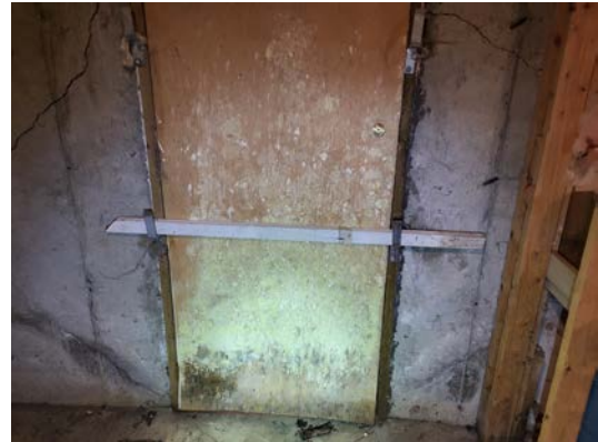
View of door to Bulk-head
