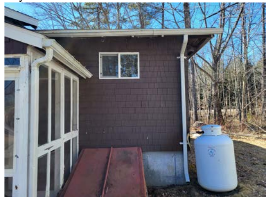
Gutters on these roof lines
