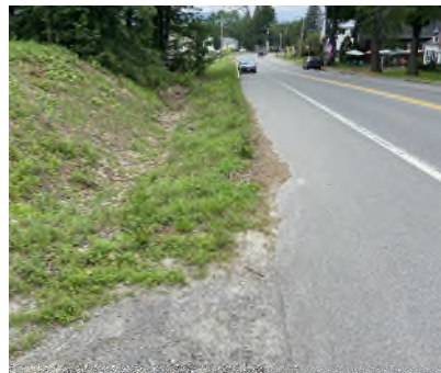
Drainage swale along Rt. 27 and Self-Storage Lot facing north
