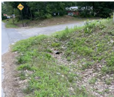
Self-Storage Lot driveway culvert and swale facing south
