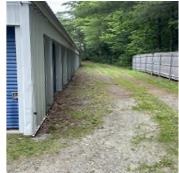
Fence along south property line
