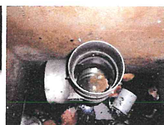
PL-68 outlet filter baffle
