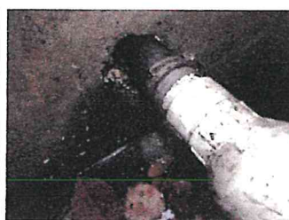
effluent is entering the lift tank from the pressure line exit hole and not baffle
