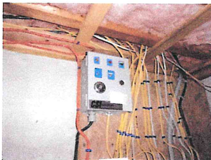
high water audible alarm box
