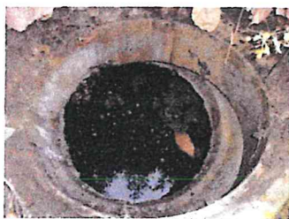
center access riser has shifted
