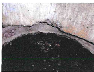
chunk of concrete missing from the bottom of the riser
